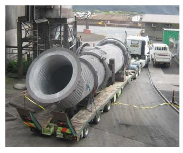
New Zealand Steel's 25 tonne gas radiation shaft waits to be lifted into place with the help of 3D computer modelling, a purpose-built, twin-hoist overhead crane, careful planning and teamwork. The project won the 2010 Crane Project of the Year.
